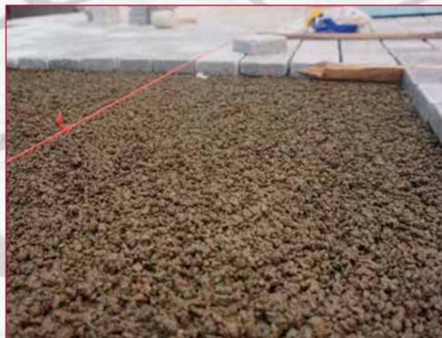
ROMEX<sup>®</sup> TRASS-BED and ADHESION ELUTRIANT
